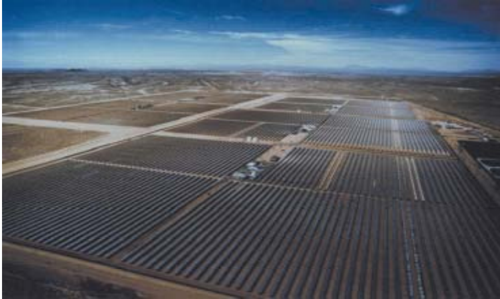
Figure 1.1 Aerial view of five, 30-MW SEGS solar plants (source: Price et al. 2002)
