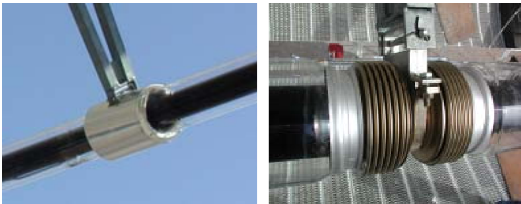
Figure 2.4 Close-up of receiver support bracket attachment to absorber tube
