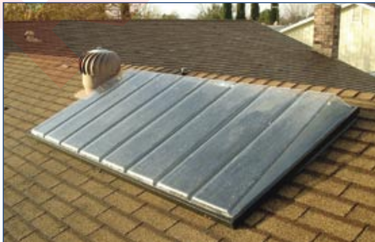
Fig. 3.3.2-1 Prototype polymer solar water heater for warm climates.
