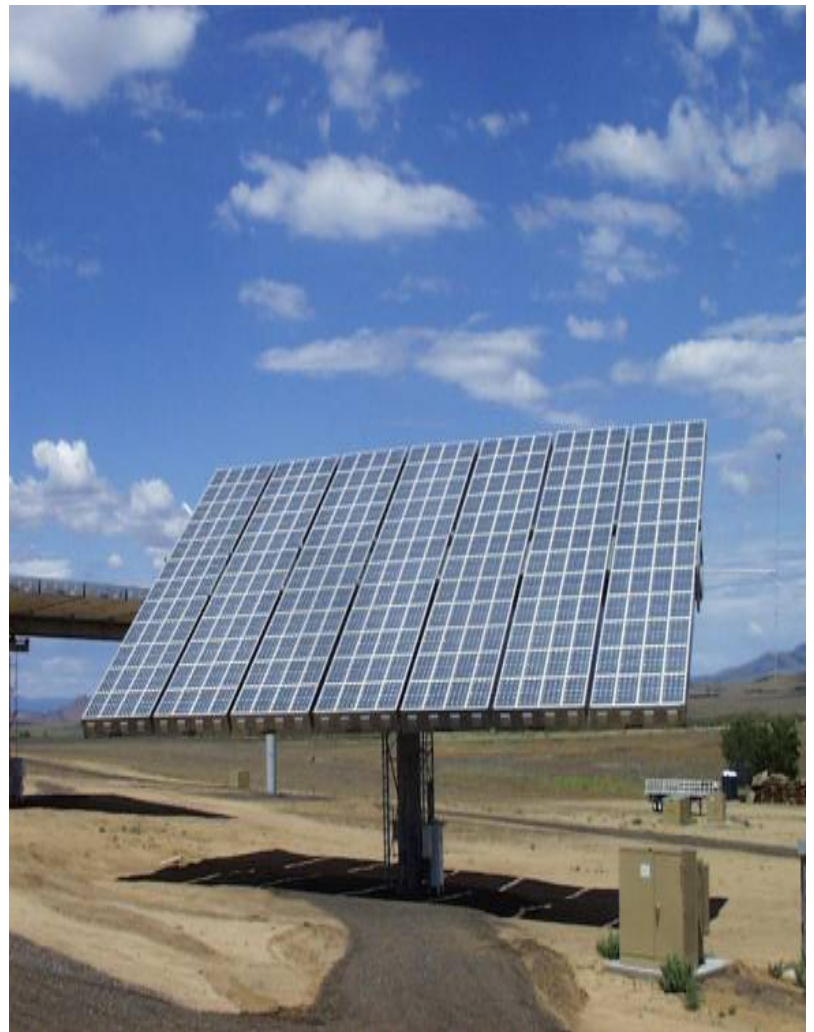
Arizona Public Service photo: Prescott 35 kW, dual axis tracking system.
