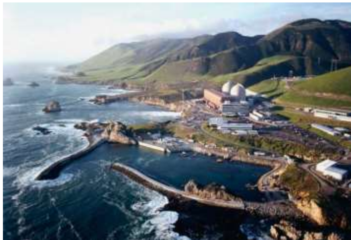
Figure 10 - East and West Breakwater and Harbor Area
