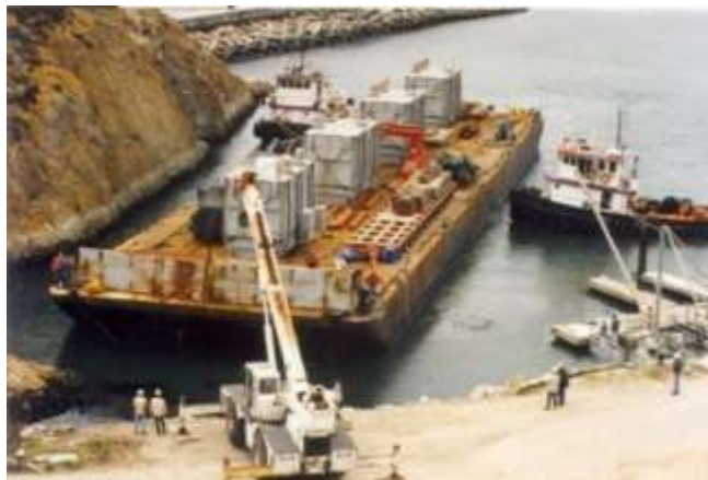
Figure 11 - Use of Barges to Bring in Materials - 1994
