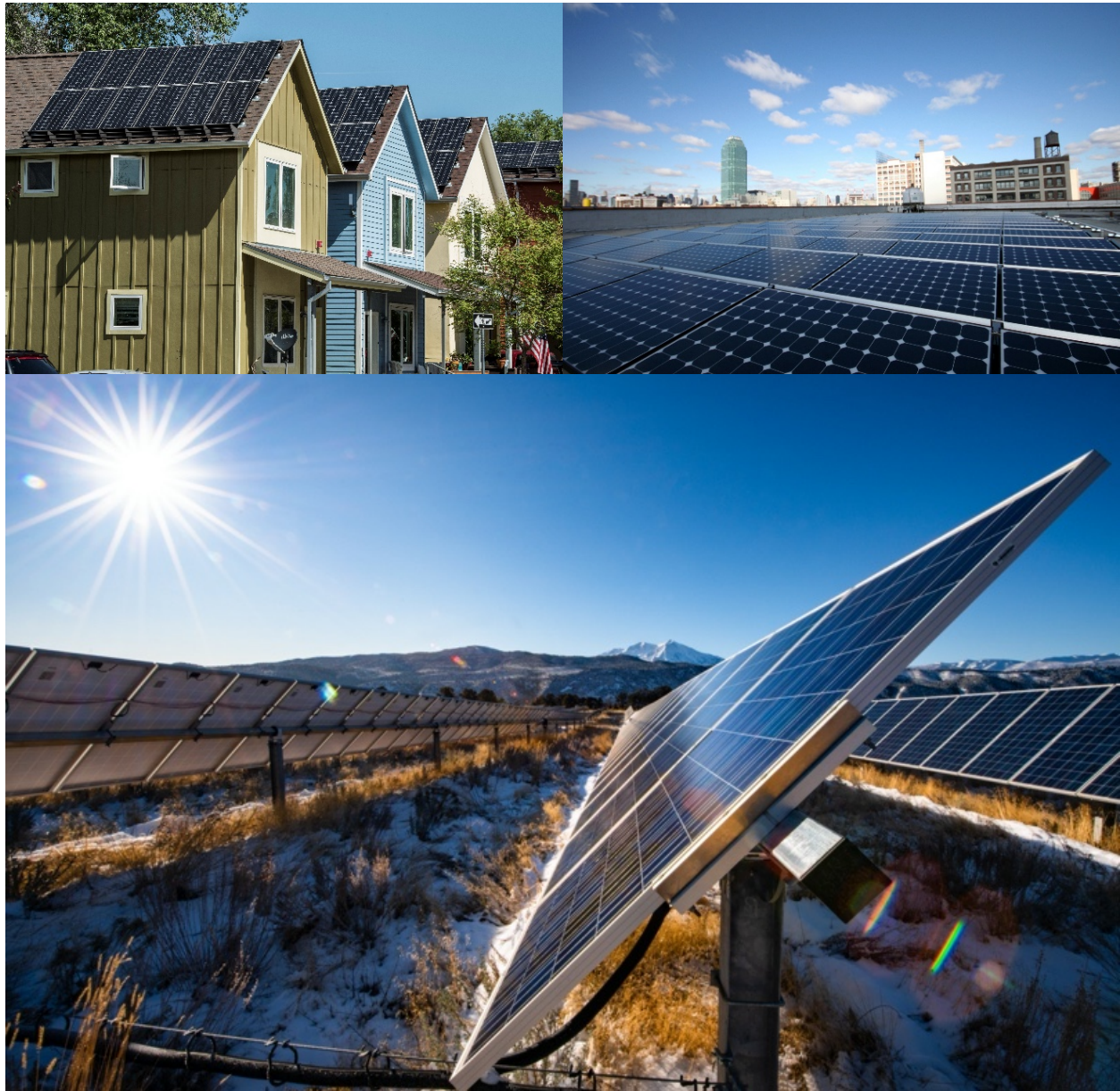
Figure 3. Residential (top left), commercial (top right), and utility-scale (bottom) PV systems
