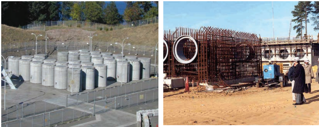
FIGURE 3.2. An example of a vertical (left) dry storage configuration of spent nuclear fuel from the decommissioned Trojan Nuclear Power Plant in Oregon. The horizontal (right) configuration, under construction, shown is from the Calvert Cliffs Nuclear Power Plant in Maryland.
