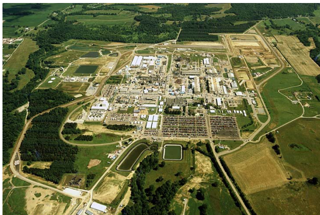
The Feed Materials Production Center (Source: U.S. DOE, 1998)
