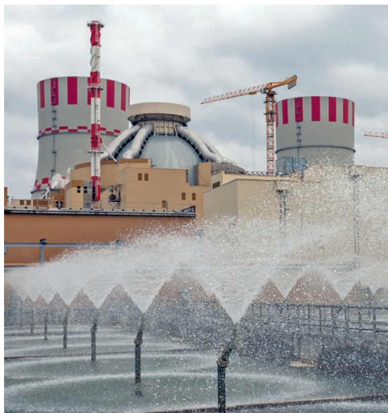
Sprinkling pool, part of the plant's cooling system (Image: Rosatom)
