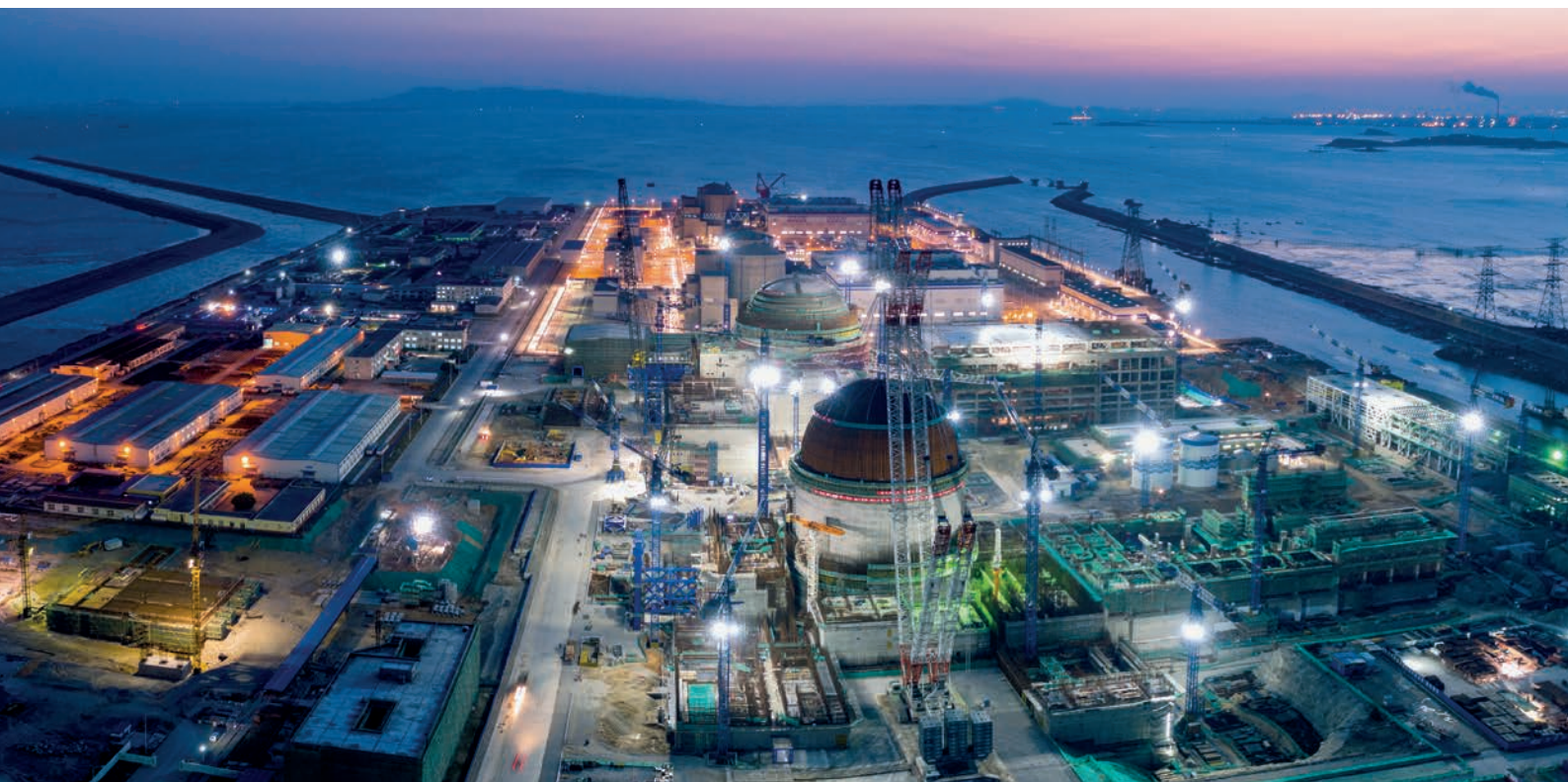
Fuqing power plant (Image: CNNC)
