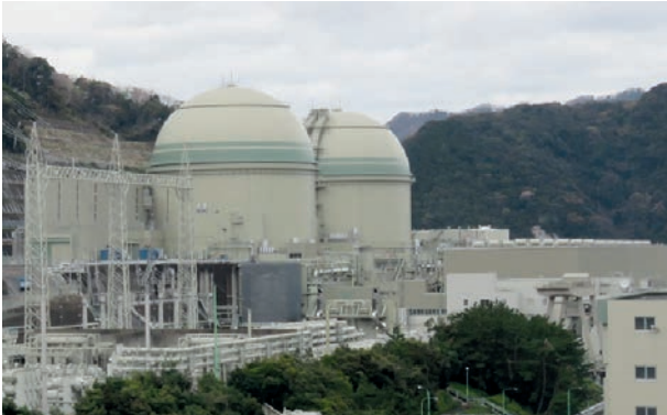
Takahama 3 and 4 (Image: Kansai Electric Power Co)
