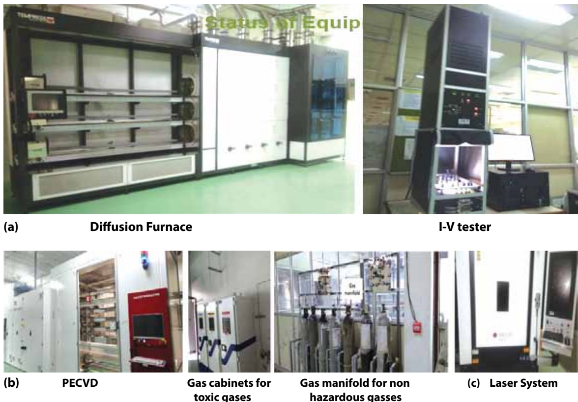
Fig. 7.14: PERC Solar cell development facility at BHEL ASSCP Gurugram
