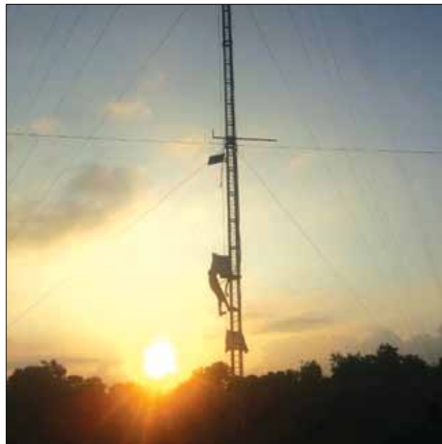
Fig. 10.18 Commissioning of 100m WMS in Gujarat
