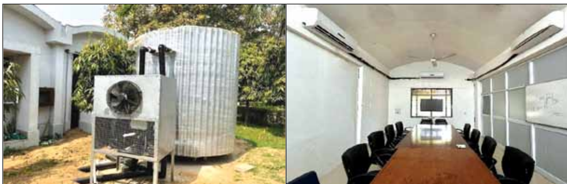
Fig 10.4: (Left) Heat pump outdoor unit with thermal storage tank and (Right) indoor unit of heat pump
