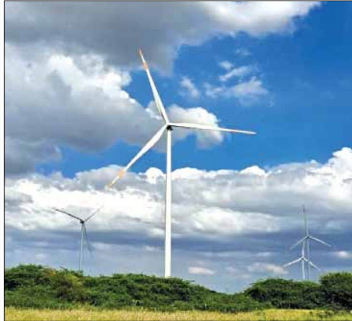
Fig. 10.32: 229.5 MW Wind project in Gujarat under SECI Wind (Tranche V) tender
