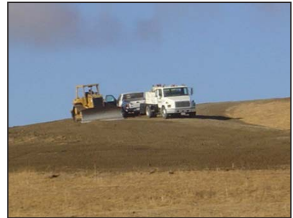
Graded area is ready for seeding
