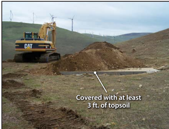
Foundation location on high slope area
