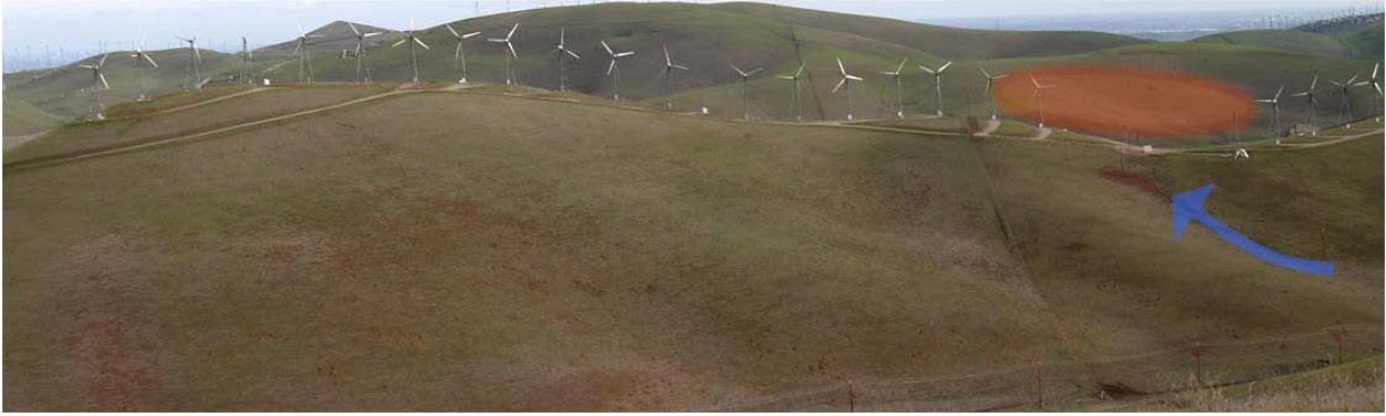
Photo 11. Turbines should not be relocated to ridge saddles, especially where declivity winds from a prevailing wind direction funnel into the saddle, as in the red zone at the right side of this photo.
