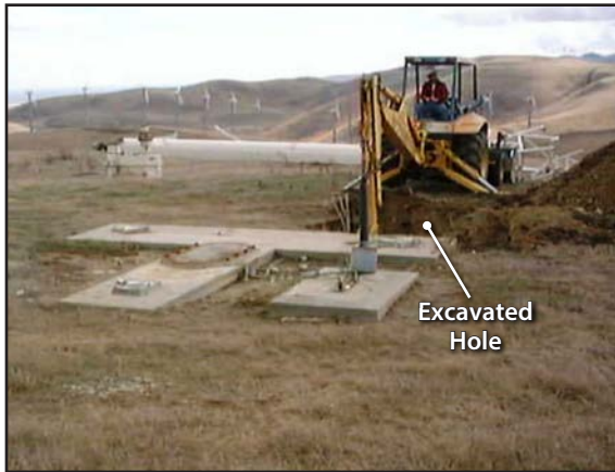
Excavation of hole adjacent to foundation
