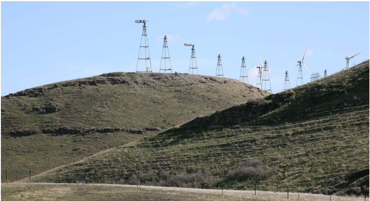
Photo 17. Derelict towers should not be put back into service where they abut steep slopes or ravines.
