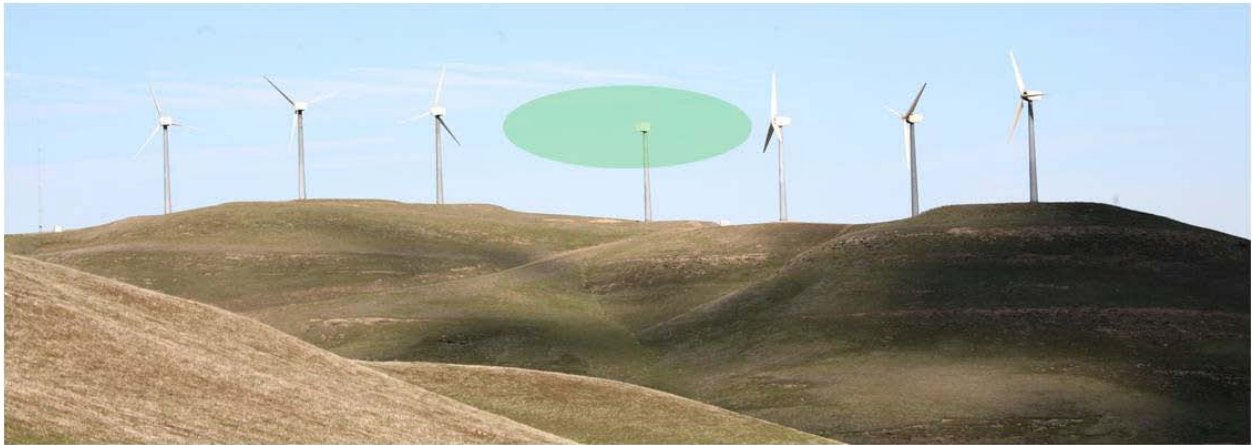
Photo 6. Turbine relocations would be relatively safer at towers interior to the turbine rows and atop a hill or ridge.
