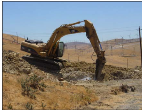
Breaking up the foundation
