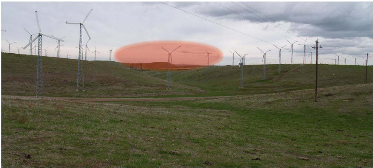
Photo 23. Wind turbines should not be relocated to towers within otherwise wide gaps between other turbines, such as seen above.
