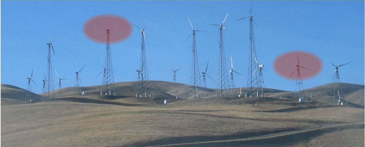
Photo 3. Turbines missing from tall towers in wind walls (e.g., red highlight at left) can create vertical and lateral gaps in turbine operations, which might be misperceived by raptors as safe perches or fly-through locations. Turbines removed from shorter towers, such as the functional one highlighted on the right, can also create vertical and lateral gaps.
