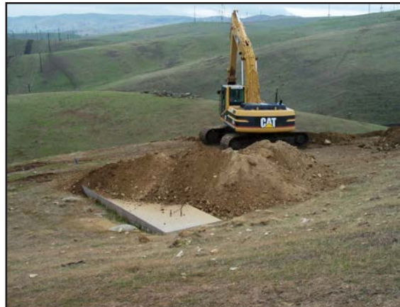
Dirt is moved from the lower bank to fill in the turbine pad area and foundation
