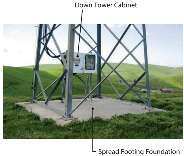
Spread Footing Foundation for Lattice Tower
