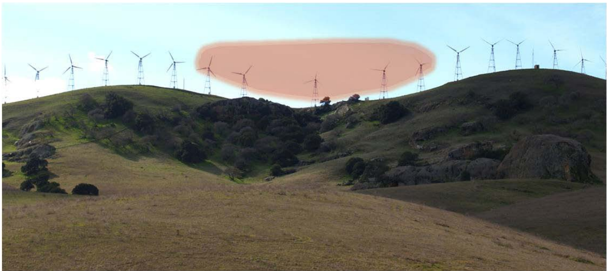
Photo 10. Turbines should not be relocated to ridge saddles, especially in a situation like above, where trees and rock formations occur nearby.
