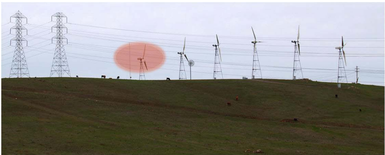
Photo 19. Avoid relocating wind turbines next to transmission towers or other perch sites.
