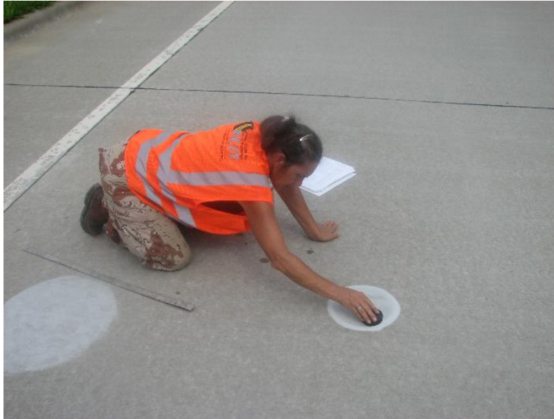
Figure 36. Sand patch testing
