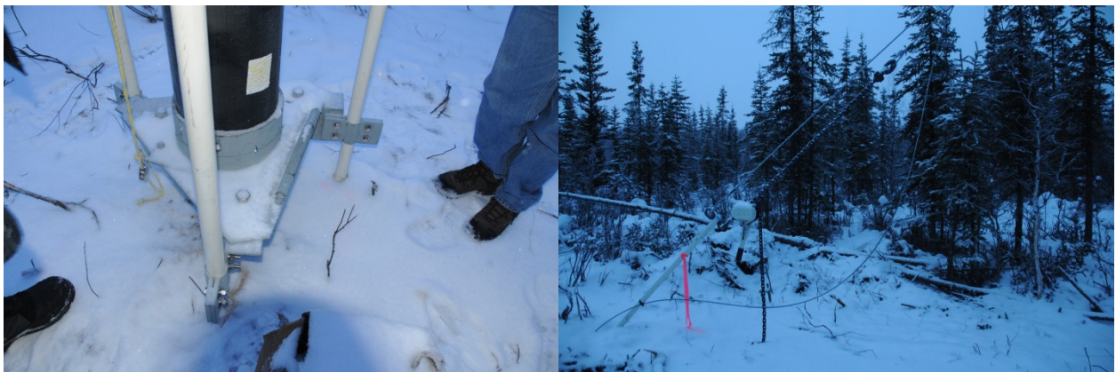
Figure 9: GFRP Pole Foundation (left) and Guy-Wire Anchor (right)
