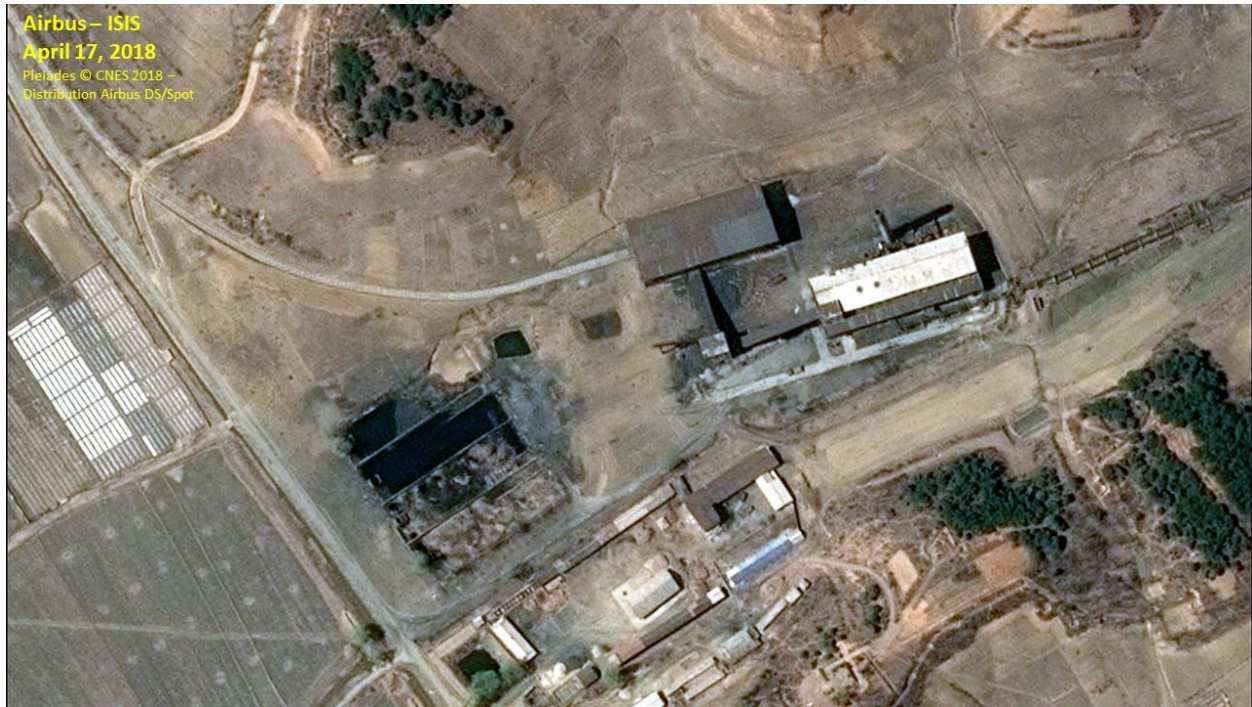
Figure 5. The coal-fired steam generation plant shows no visible signs of operation. Operation would indicate the operation of the nearby Radiochemical Laboratory.
