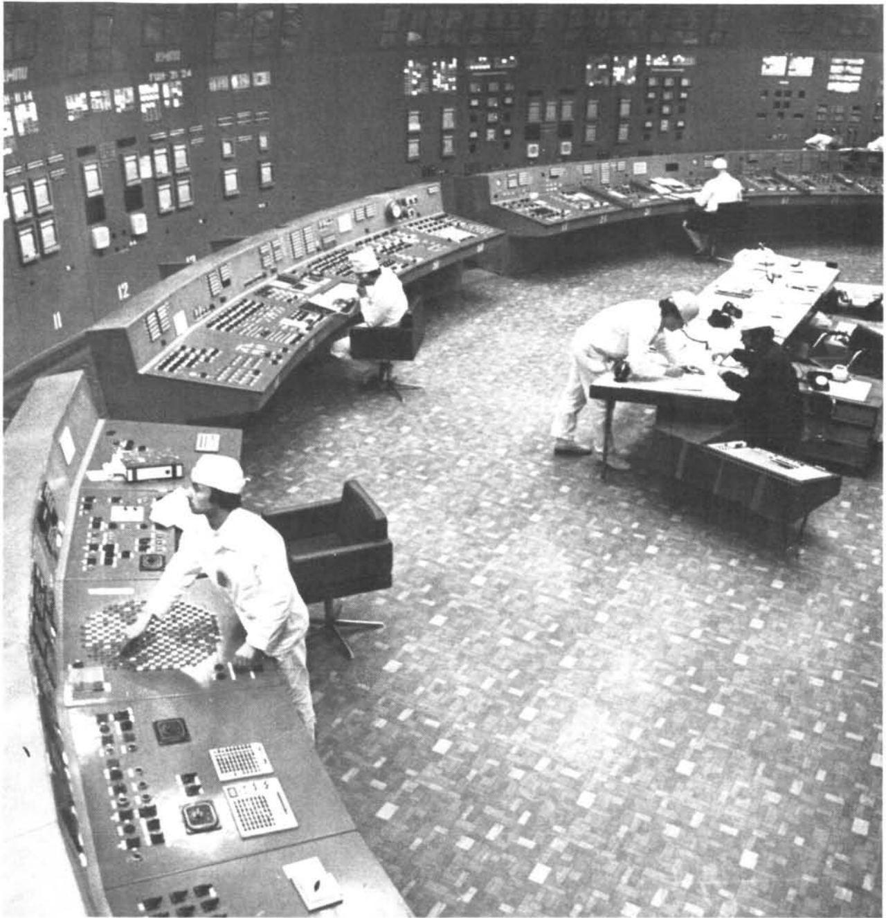
The control-room of the 1000 MW RBMK Smolenskaya nuclear power plant, one of the most modern power reactors in the Soviet Union.
