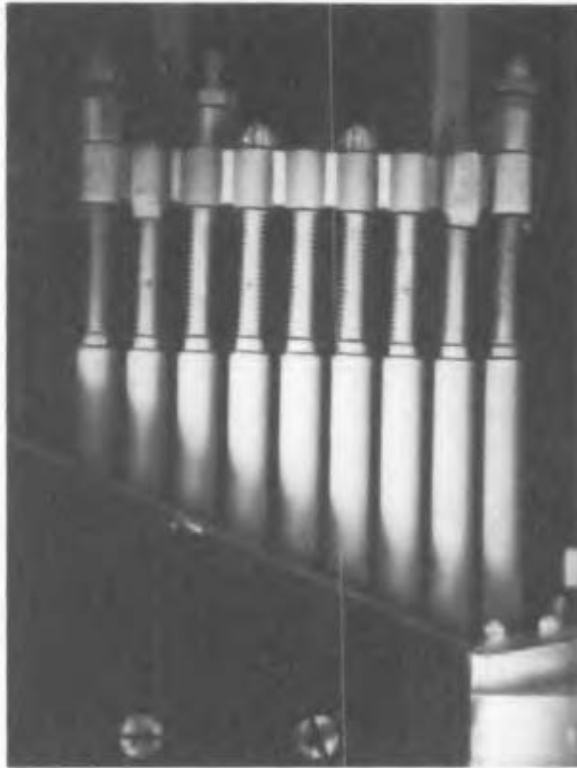
FIG.28. Visual underwater inspection of upper end of BWR fuel assembly (stainless steel tie plate and Zircaloy-clad fuel rods).
