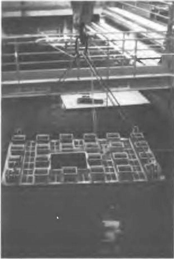
FIG.8a. Top view of SS rack being removed from a PWR spent fuel pool (rack dimensions: 295 cm X 195 cm). Early design; does not utilize neutron absorbers.
