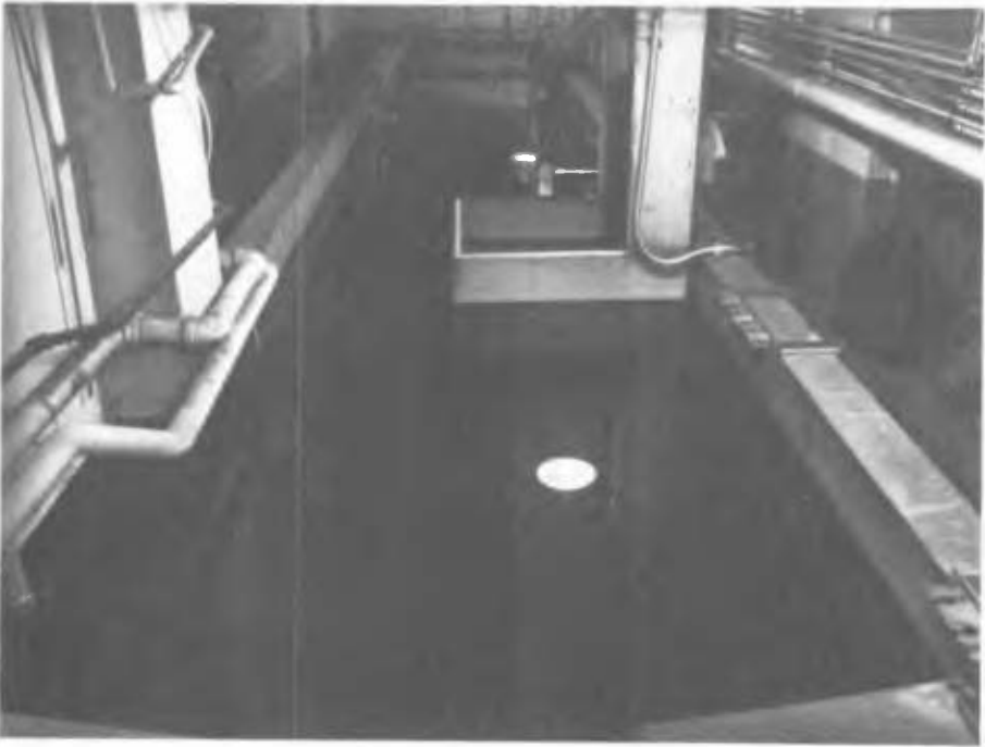
FIG.1. X-10 research reactor fuel pool at Oak Ridge National Laboratory, TN, USA. The X-10 is the site of the world's first storage of irradiated nuclear fuel. The first fuel discharge was in November 1943 and the reactor operated until 1963. The spent fuel pool still stores irradiated materials (1980) and is also used for intermittent storage of fuel.
