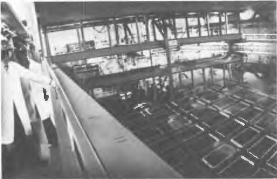
FIG.5. PHWR pool at Pickering reactor, Toronto, Canada. (Fuel stored in stainless steel trays.)
