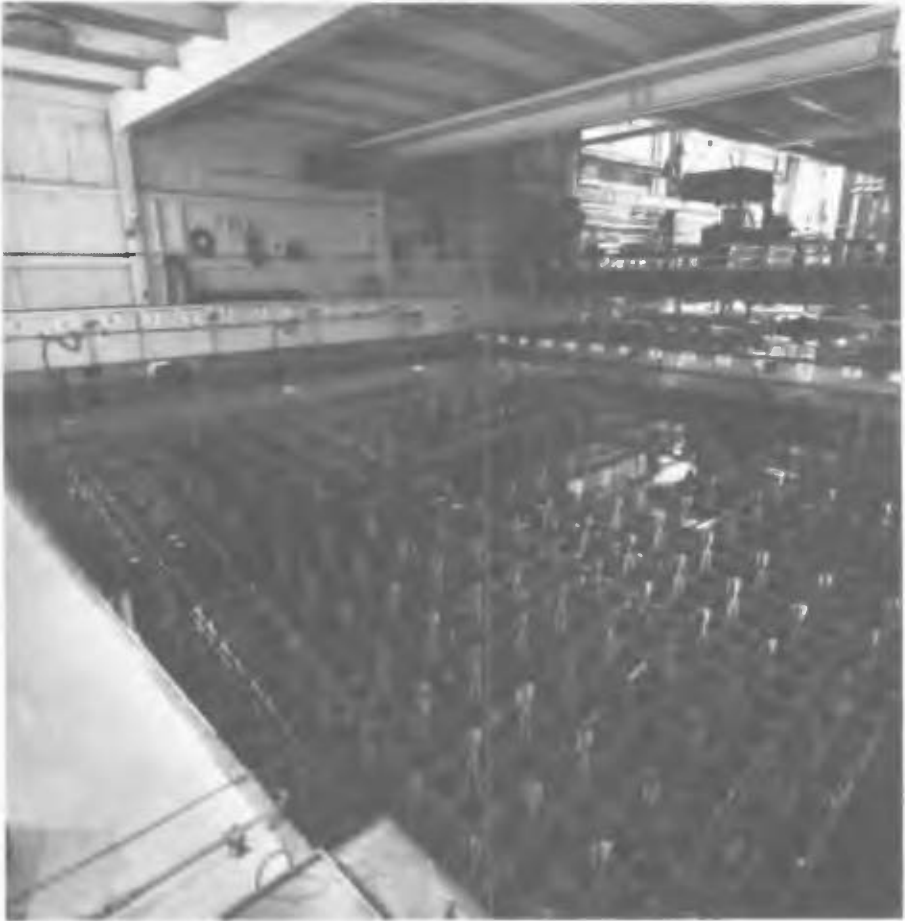
FIG.6. AFR pool at General Electric Co., Morris, IL, USA (Fuel stored in stainless steel baskets.)
