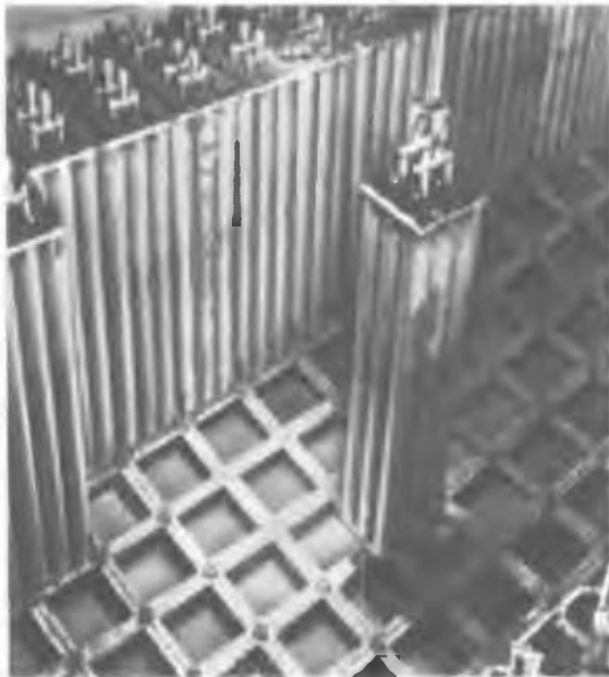
FIG.11b. G.E. Morris operation pool, Morris, IL, USA. Fully loaded BWR spent fuel storage basket (stainless steel) being transported to a pool storage location; water depth: 8.7 m.
