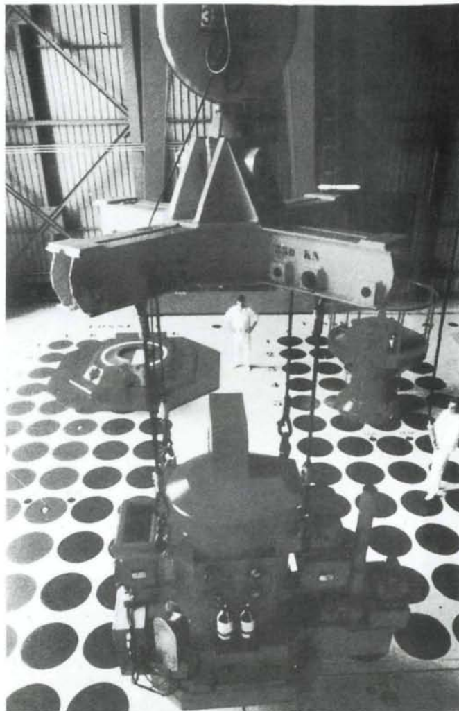
At the Marcoule facility in France, containers of vitrified high-level waste are transferred to air-cooled shafts for interim storage. (Credit: ANDRA)
