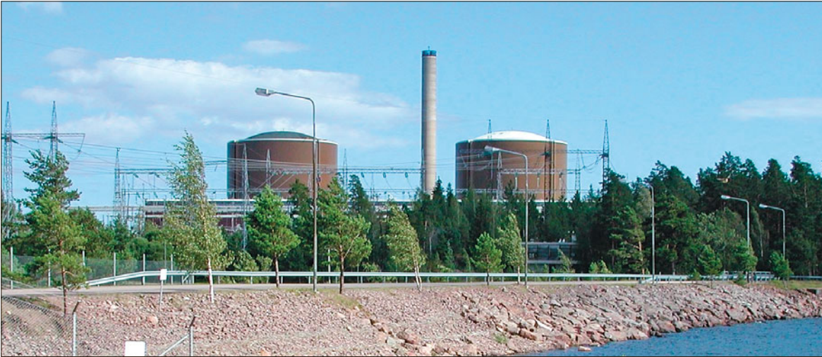
09 Loviisa power plant on the island of Hästholmen in Loviisa. Source: Fortum.
