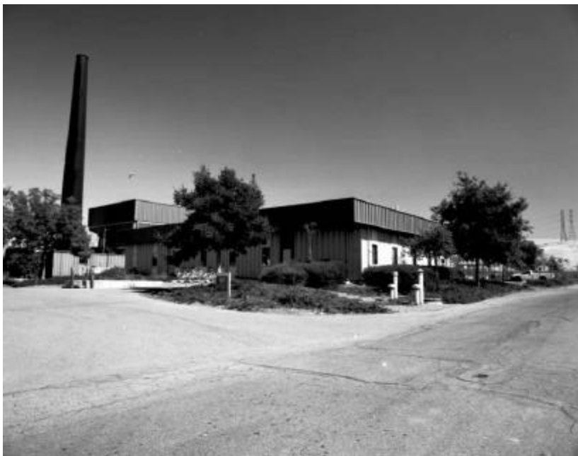
Figure 5. The Chemical and Radiation Detection Laboratory. 16
