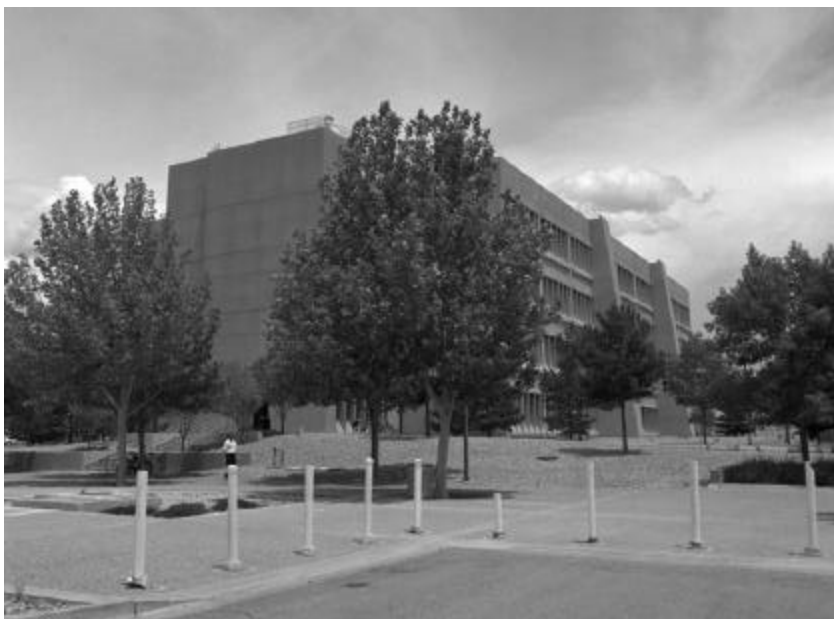
Figure 9. Building 890 at SNL/NM. 20
