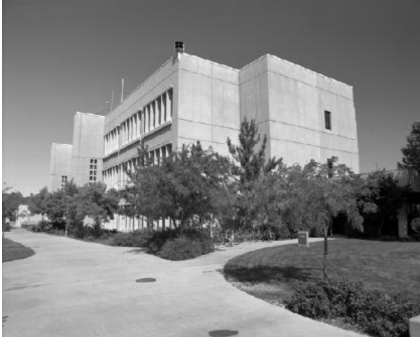
Figure 8. Building 910 at SNL/CA. 19
