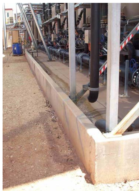
Figure 15 Example of concrete bunding, at Beverley process plant
