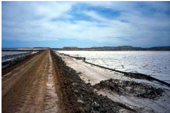
Figure 10 Example of tailings storage facilities (Provided by Graham Taylor)
