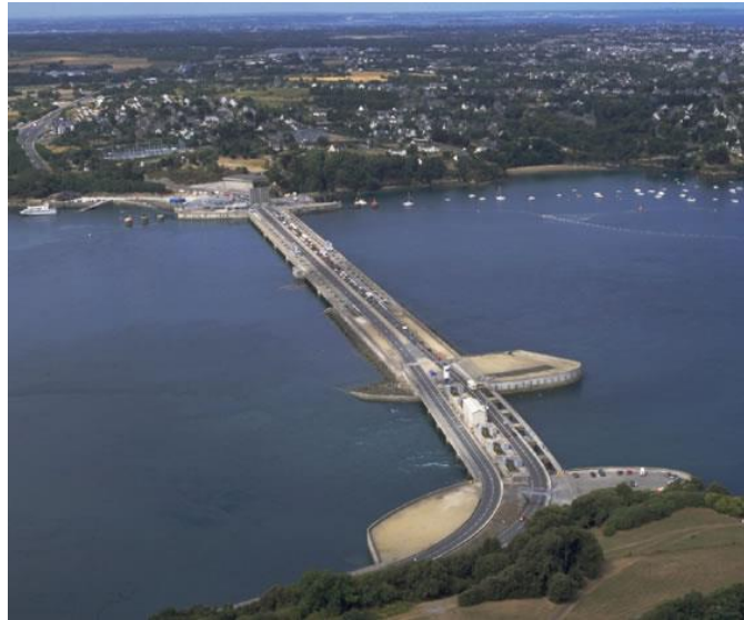
FIGURE 7: LA RANCE TIDAL RANGE BARRAGE IN FRANCE
