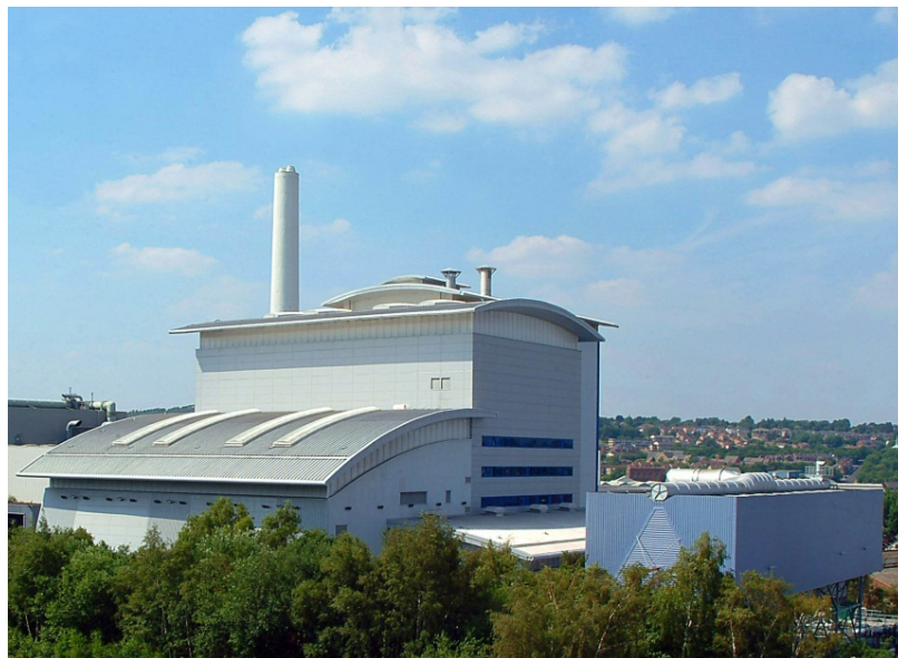
Sheffield Energy from Waste plant. Image courtesy of Veolia Environmental Services (UK) PLC.
