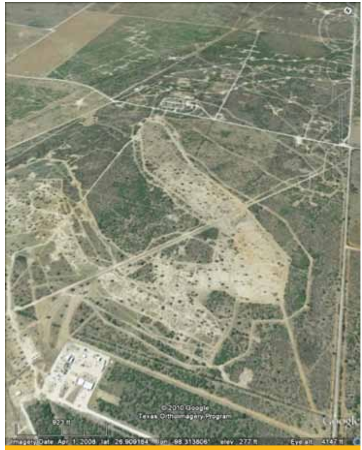
Figure 18: A portion of Mestena Uranium's Alta Mesa in-situ leach facility in Brooks County, Texas. The processing plant is at lower left. Source: Google Earth.
