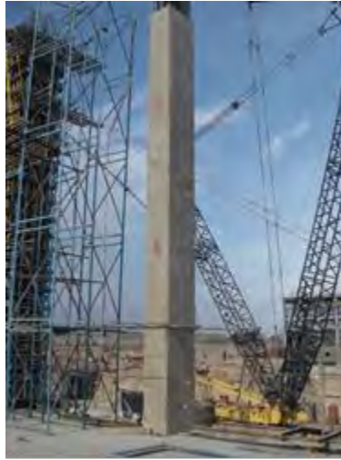
Figure2. A 10 m high column of turbine building, RAPP-5&6 constructed with SCC
