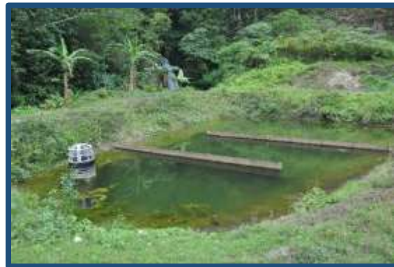
Sediment Control at Faga'alu Quarry
