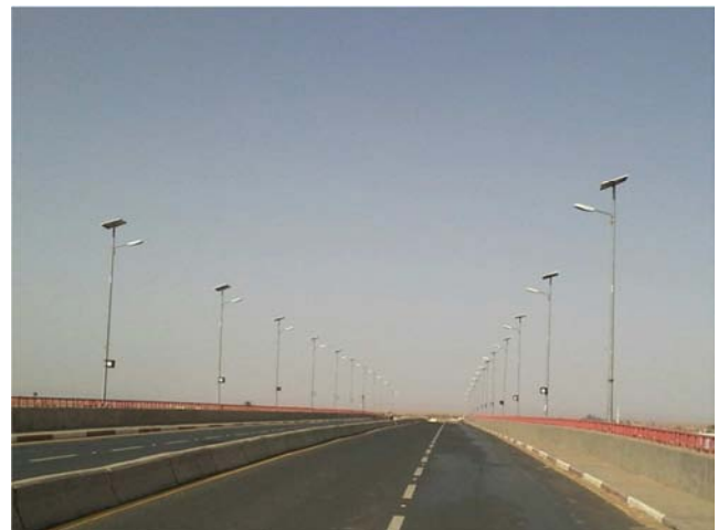
Figure 7. Solar lighting system of Aldebba- Argi Bridge.
