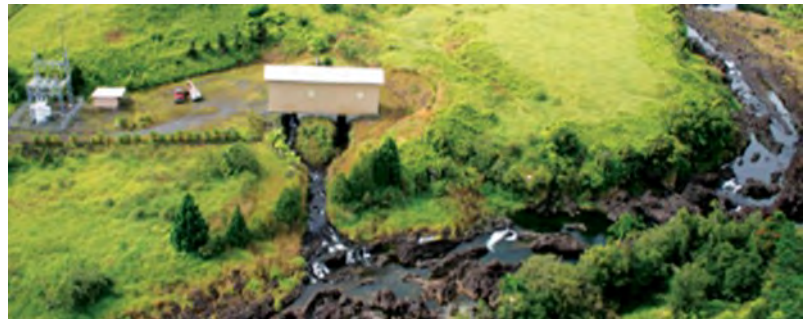
Wailuku River Hydroelectric Power Plant, 11 MW, Hilo, Hawaii
