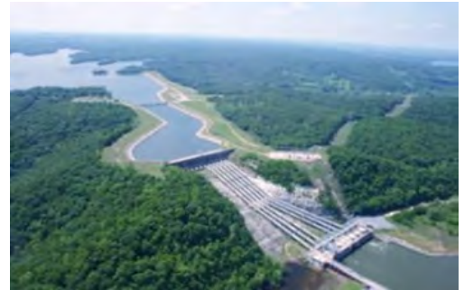
Grand River Dam Authority (GRDA) Salina Pumped-Storage Project, Oklahoma
