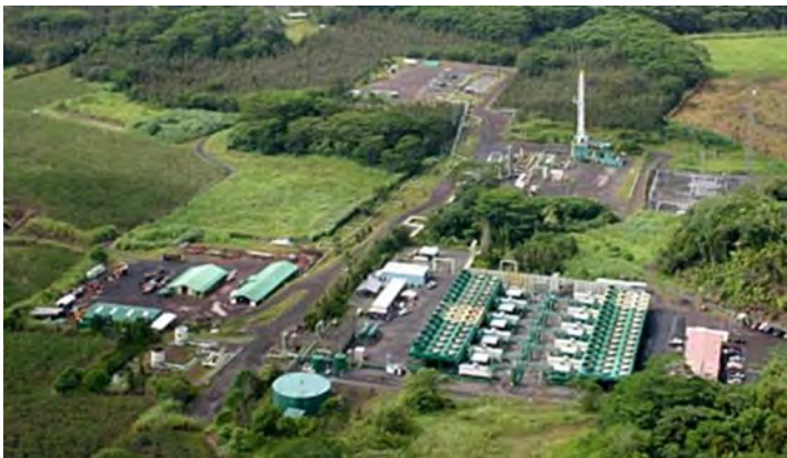
Puna Geothermal Venture Power Plant, Paho, Hawaii Island
