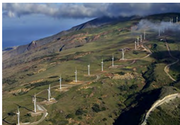
Kaheawa Wind Power I, 30 MW, Maui
