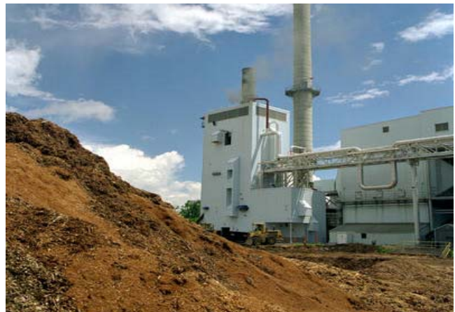
Biomass Conversion Plant
