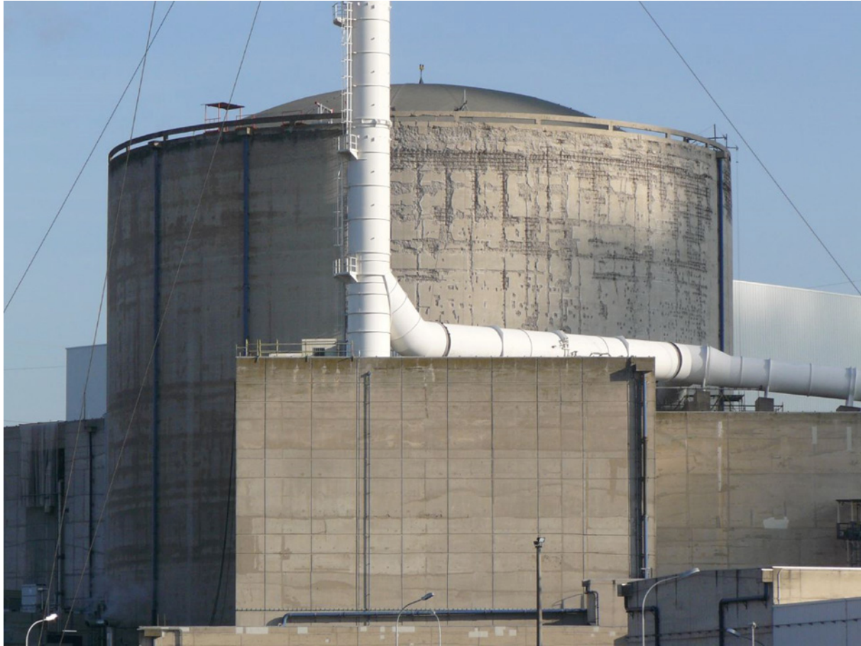
Figure 1.8: – Ageing damaged outside wall of the reactor building at the Belgian nuclear power plant Tihange. (© Alain Vincent/Greenpeace)
