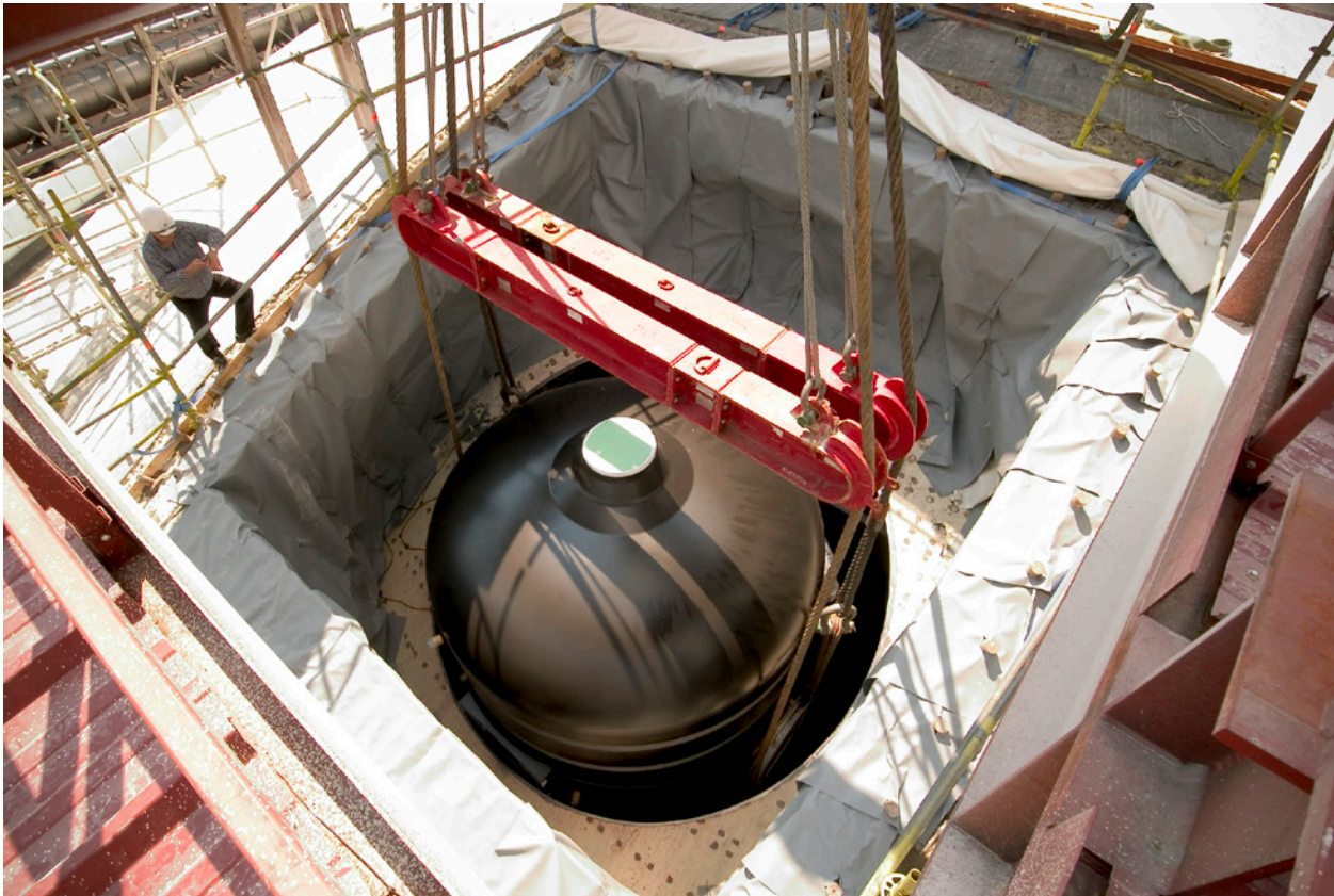
Figure 1.5 – Steam generator replacement through a hole cut into the containment at the Belgian nuclear power plant Doel 2, 2004. (© electrabel)
