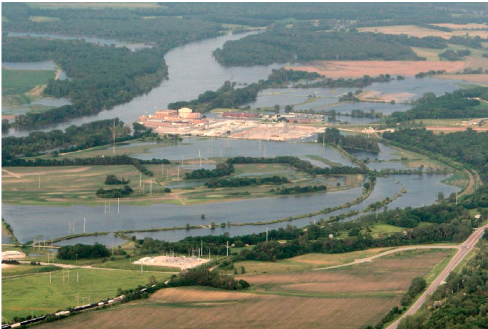
Figure 1.13 – Flooding at Fort Calhoun nuclear power plant, United States, 2011.
