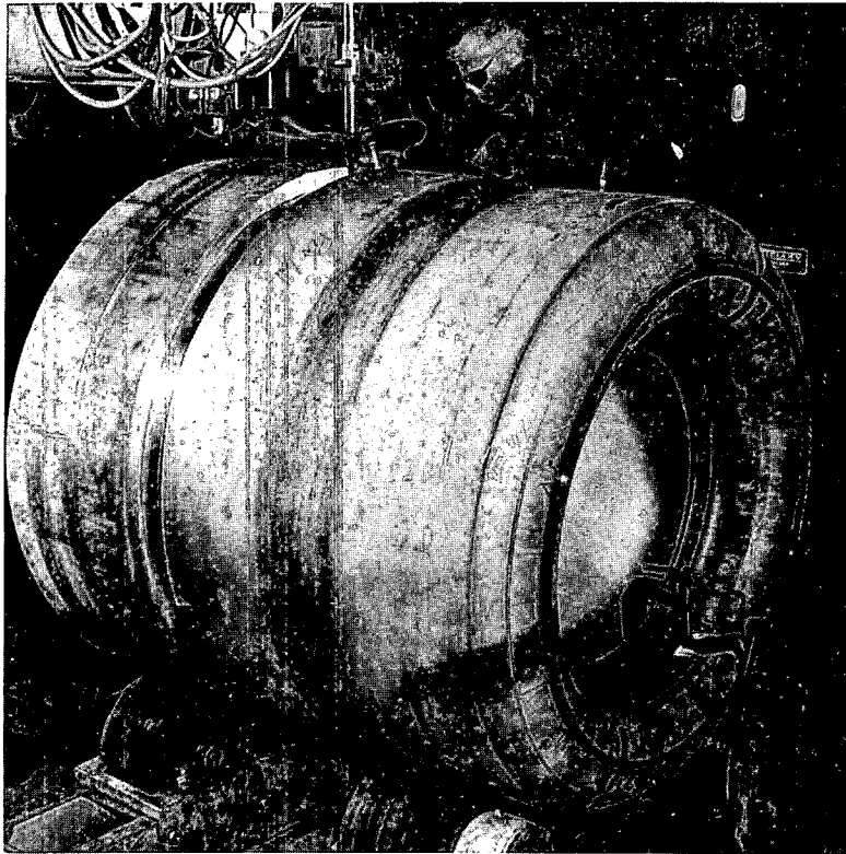
FIGURE 9. Welding of the KIWI B reactor vessel by the tungsten Inert Gas - Cold Wire Feed Process.
