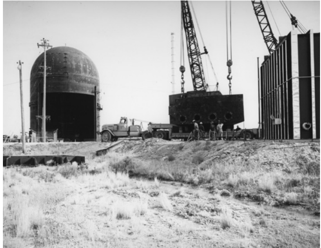
LOFT reactor under construction, 1969.
