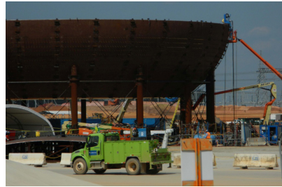
A containment vessel under construction at a nuclear power plant site.
