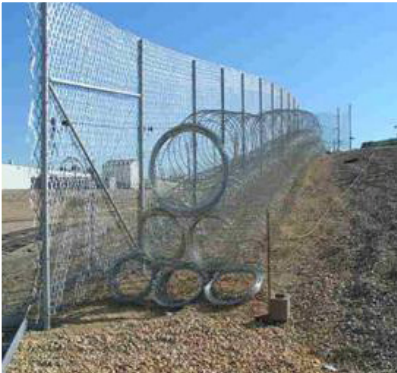
Barriers are part of the physical protection system used by operating reactors to defend against the DBT.
