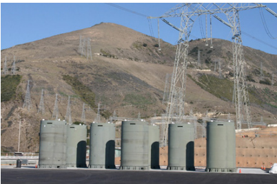
Independent spent fuel storage installations store spent fuel safely and securely.
