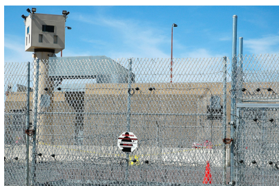
NRC licensees have measures that limit the exposure of security personnel to possible attack, including the incorporation of bullet-resisting protected positions that provide protection against the DBT.
