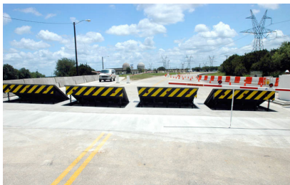
Vehicle barriers are part of the physical protection system used by some nuclear facilities.
