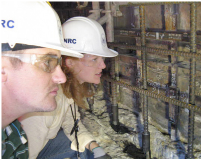
An NRC inspector gathers information at a nuclear power plant.
