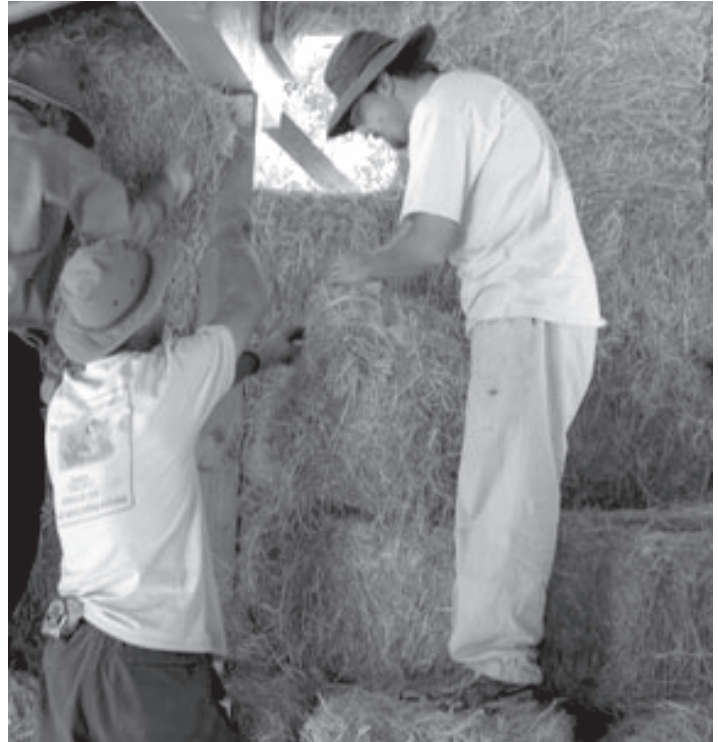
Figure 1: Constructing an infill strawbale building.
