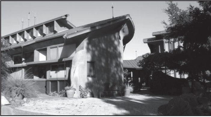
Figure 2: Passive solar strawbale building design in Santa Margarita, California.
