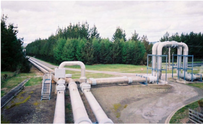
Figure 14 – Geothermal power generation is compatible with other land uses, as demonstrated by steam pipelines for a plant in Ohaaki, New Zealand, that run through land used for grazing and agriforestry. (Credit: Evan Hughes for EPRI)
