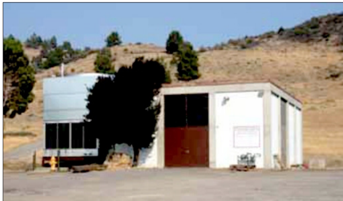
Figure 4. Power house with water cooling tower [2].
