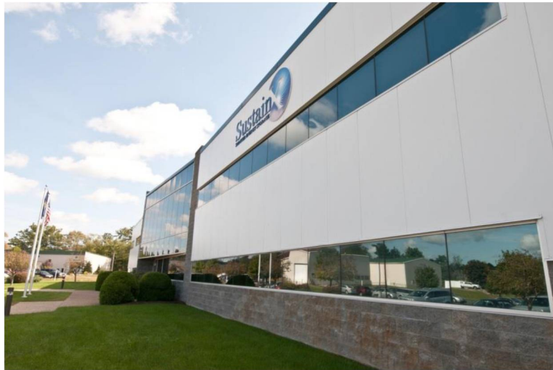
Figure 1: SustainX facility in Seabrook, New Hampshire
