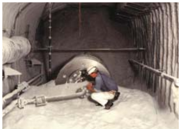
A long-term test of the behaviour of a non-radioactive, simulated high-level waste container in an experimental gallery in a mine in a deep salt formation in Germany. The container can be seen as crushed rock salt is being excavated from around it, after the test (courtesy DBE).
