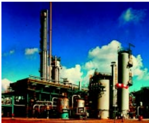
Ammonia Unit. Netherlands. (Hydro Agri Europe)
