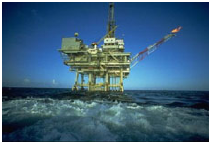
Figure 2. Offshore Template Platform
