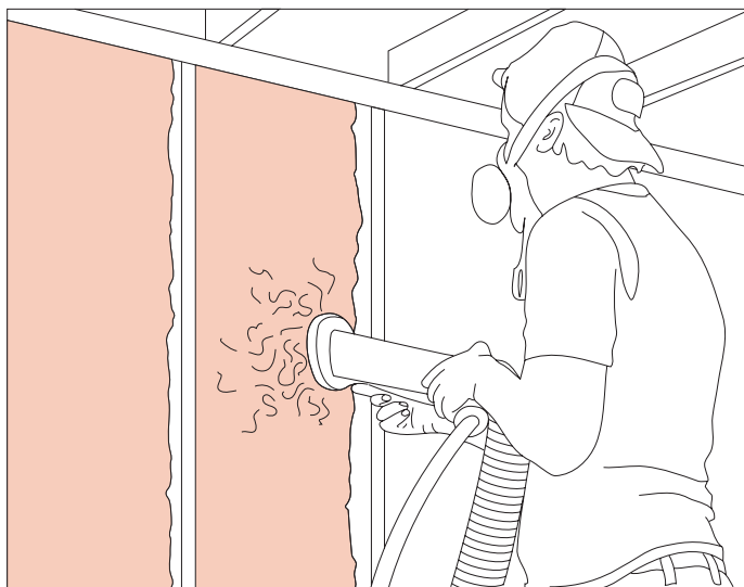
Figure 3-4 - Several types of insulation can be applied as a liquid or wet slurry. These "spray-applied" insulation materials are used mostly in new construction of walls, but some contractors use them in attics for both new construction and retrofits.
