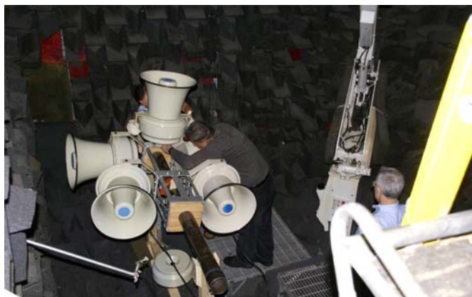
New sirens are being installed at Indian Point.
