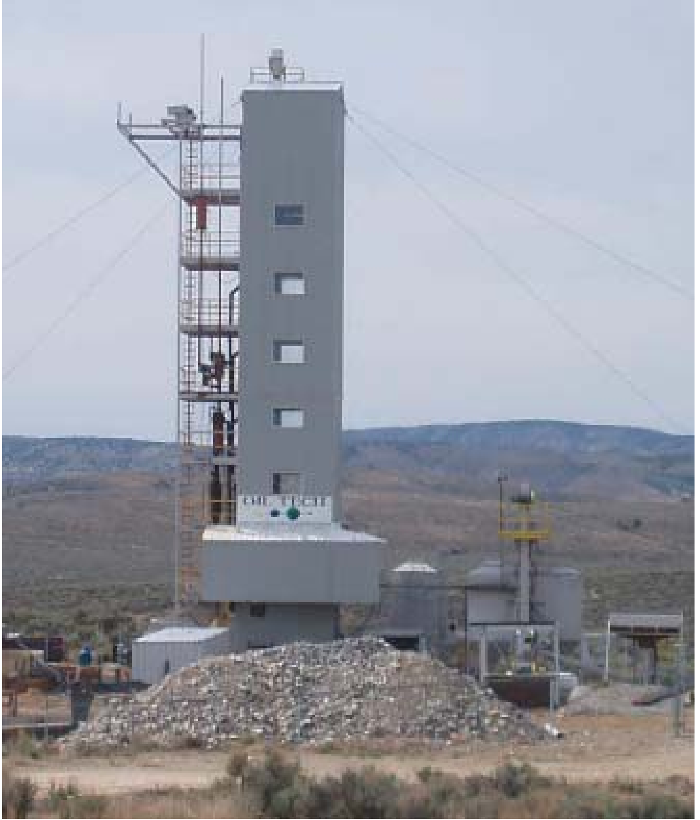
Millennium Synfuels / Oil-Tech Retort Pilot Plant – Near Vernal, Utah (2006)
