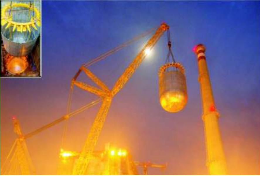
Erection of Main Vessel of Prototype Fast Breeder Reactor
