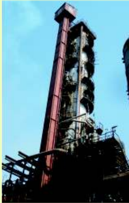
A column at HPCL, Mumbai
