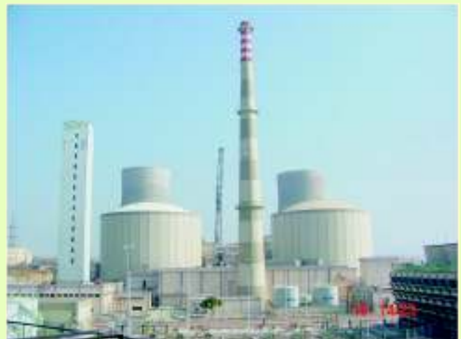
Rajasthan Atomic Power Project -5&6 Main Plant View
