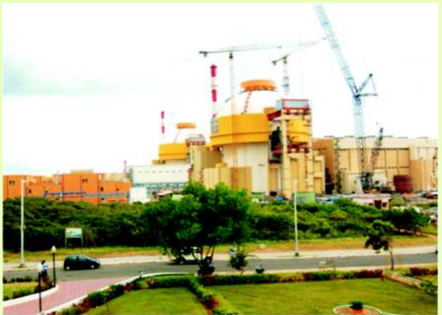
Kudankulam Nuclear Power Project - 1&2
