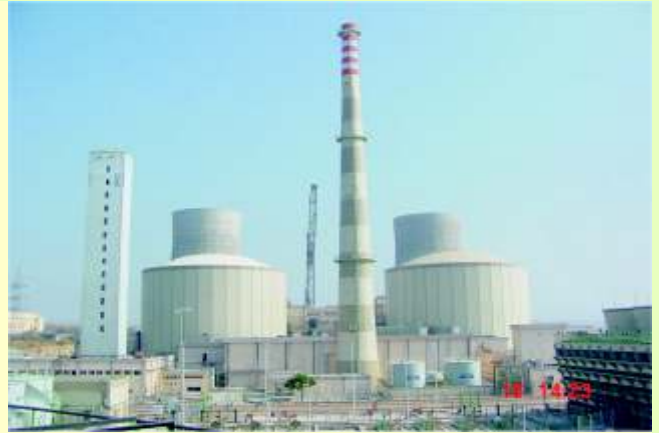
RAPP-5&6 Main Plant View
