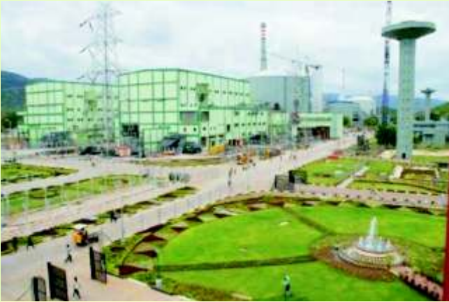
Kaiga-3&4 Main Plant from North-East
