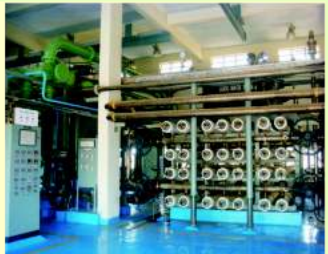
Hybrid Nuclear Desalination Demonstration Plant (NDDP) at Kalpakkam. The plant is based on MSF-RO technology
