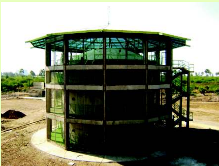
Containment Model construction completed at Tarapur
