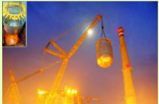
Erection of the Main Vessel of the Prototype Fast Breeder Reactor
