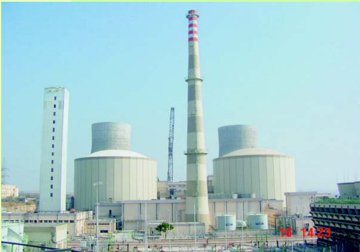
Rajasthan Atomic Power Project-5&6 Main Plant View
