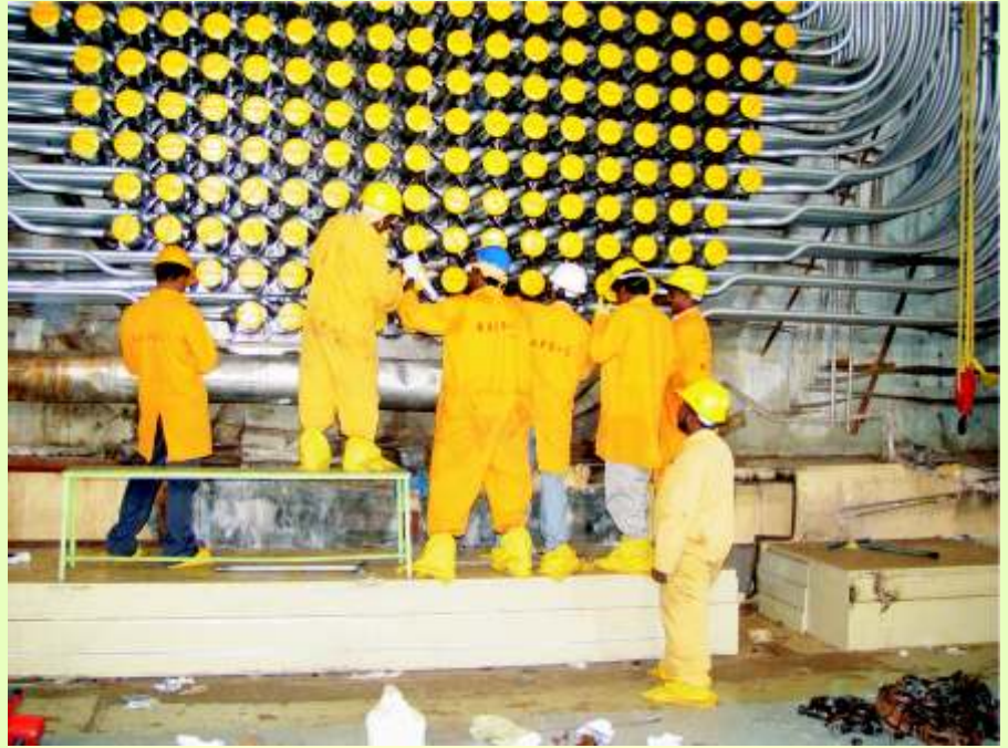
Enmasse Coolant Channel Replacement activities at KAPS-1
