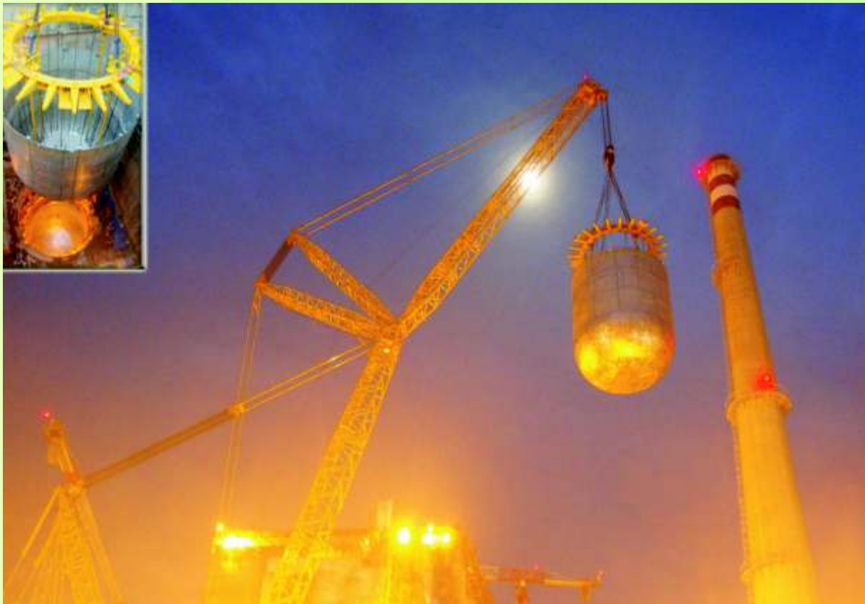
Prototype Fast Breeder Reactor's Main Vessel Erection (Bhavini)
