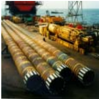
Figure 7 – Driven piles [12]
