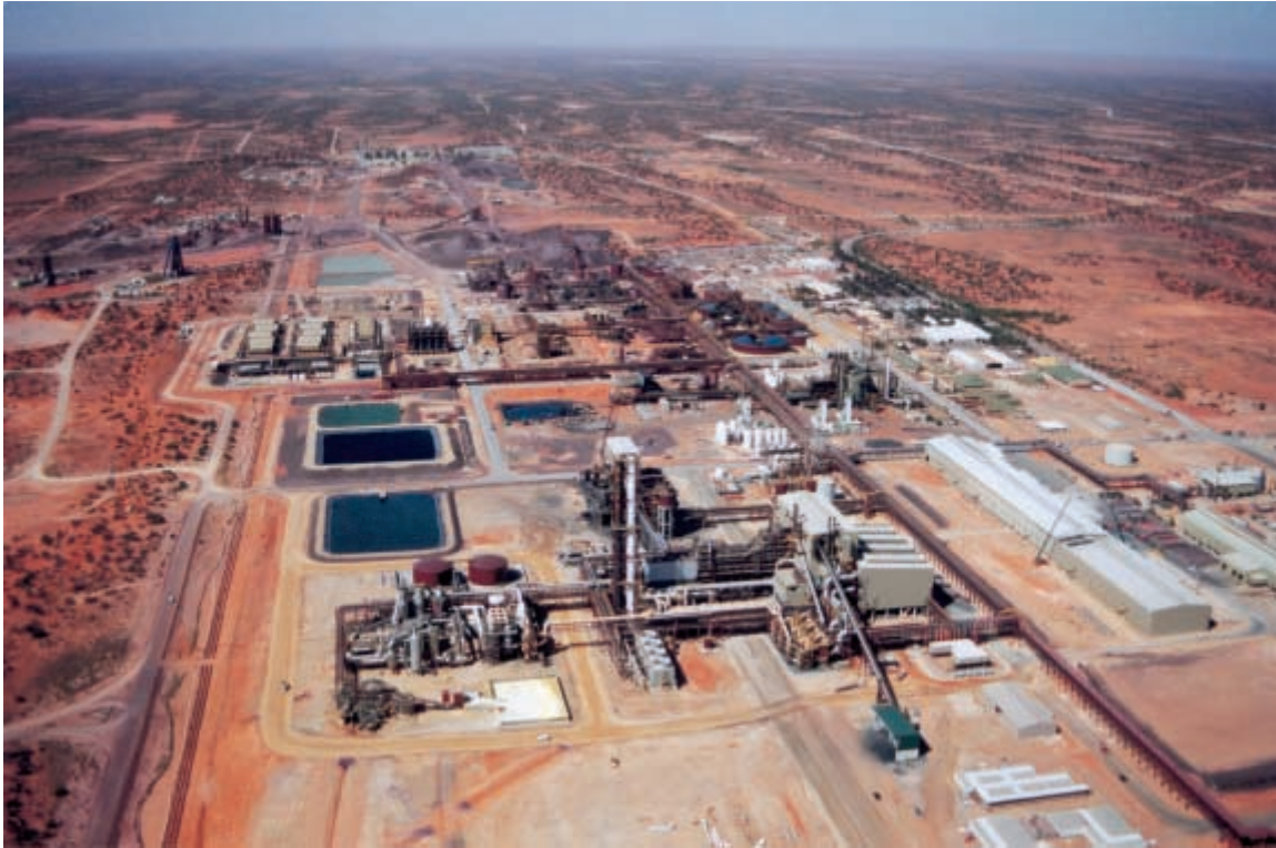
FIG. 35. Olympic Dam copper–uranium–gold mine–mill–smelter complex, South Australia. The headframes for the underground mine are near the left-hand side of the picture.
