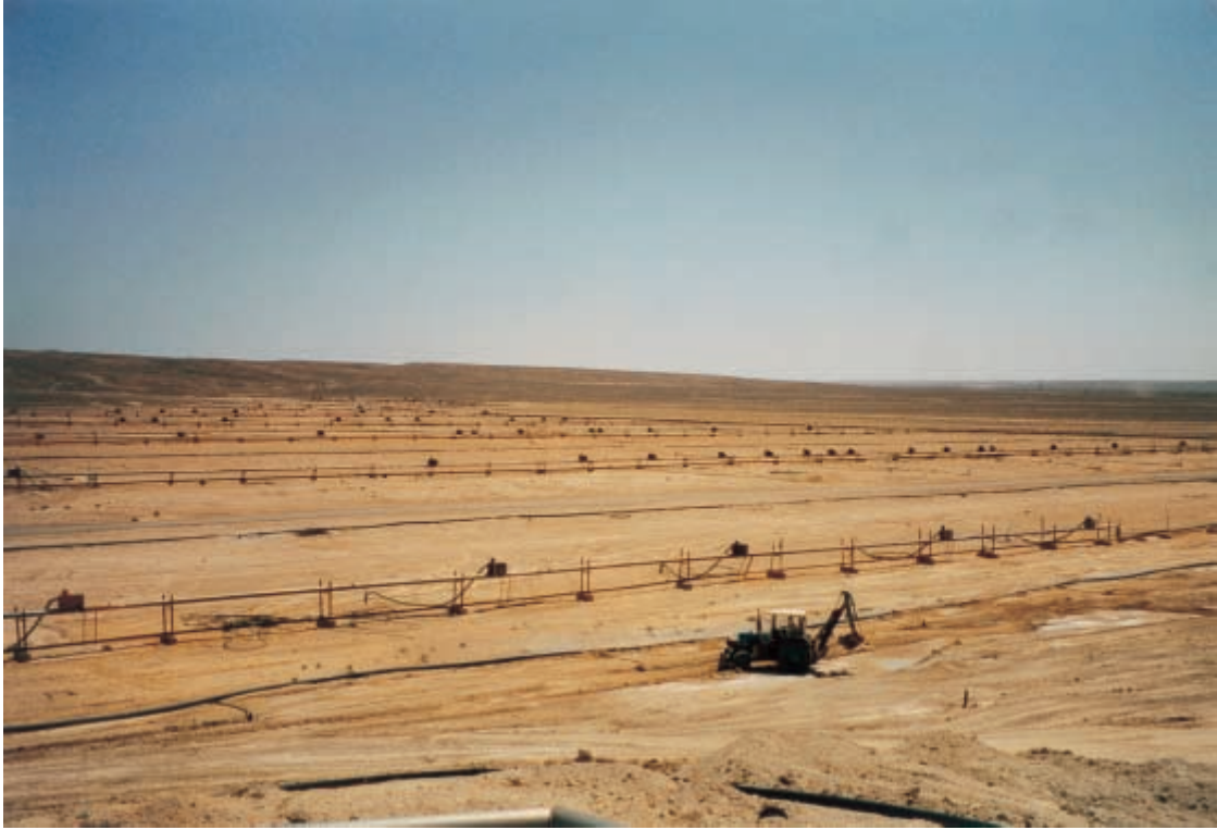
FIG. 32(a). ISL wellfield, Zarafshan, Uzbekistan. Alternating rows of injection and production wells.
