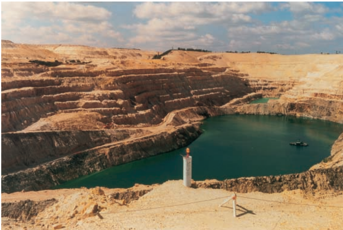
FIG. 31. Deilmann tailings management facility, Key Lake, Saskatchewan, Canada.
