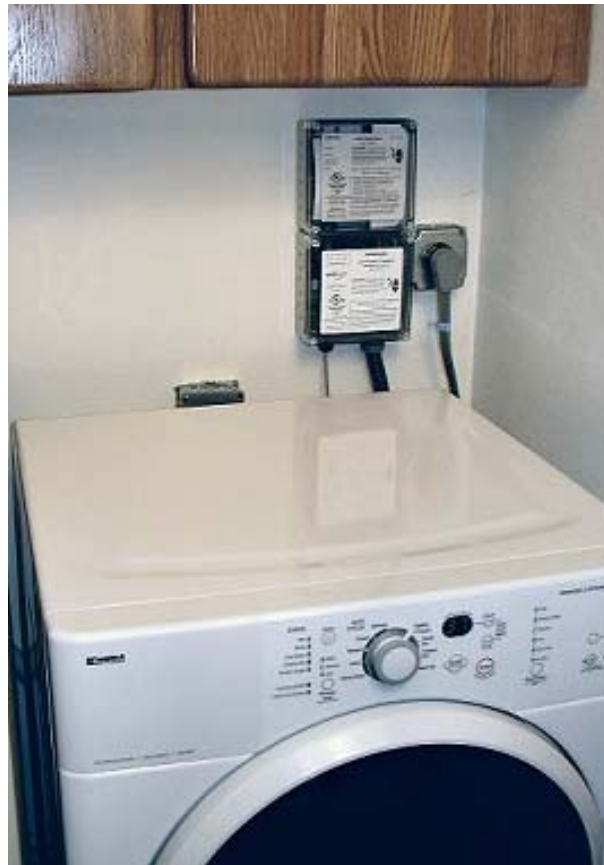
Figure 3.2. Project Sears Kenmore HE 2 Dryer and Load Control Module in a Participating Home
