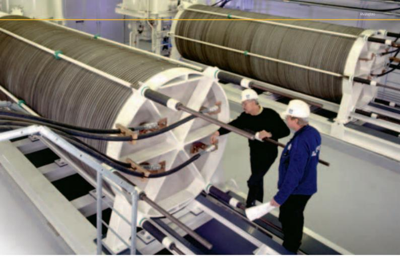
The atmospheric series electrolysers are competitively offered where hydrogen production volumes above  $50 \text{ Nm}^3/\text{h}$  are required. Our largest single skid mounted electrolyser unit has a production capacity of  $485 \text{ Nm}^3/\text{h}$ . Larger volumes are produced by simply adding more cells or additional units.
