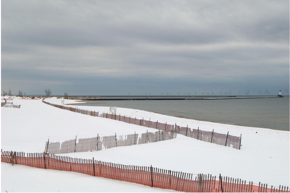
Snapshot Ludington (South viewpoint angle): 500 megawatts
