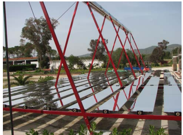
Figure 5.10 PSE Fresnel process heat collector powering a NH 3 /H 2 O absorption chillers (2008, Grombalia, Tunisia)
