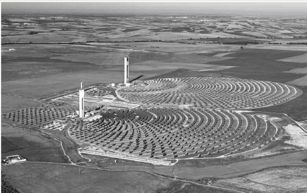
PS10 and PS20, two solar tower power systems, together generate 31 megawatts outside of Seville, Spain
